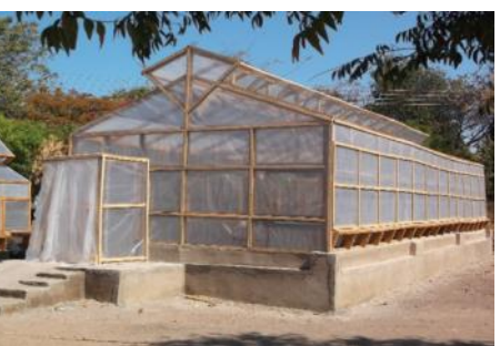
Completed solar tent fish drying unit.
