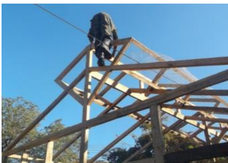
Cover the framework with chicken wire.
