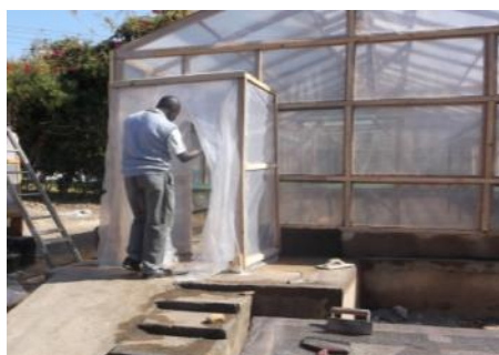
Finish by constructing a fly screening unit at the entrance/door.
