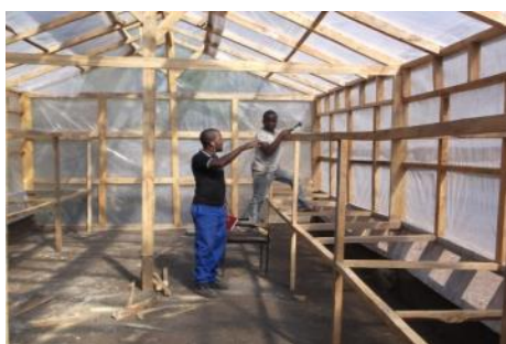
In the interior, build drying racks using 2"x 2" planks, chicken wire, and plastic gauze.
