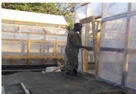
Adjust the door to the main frame.
