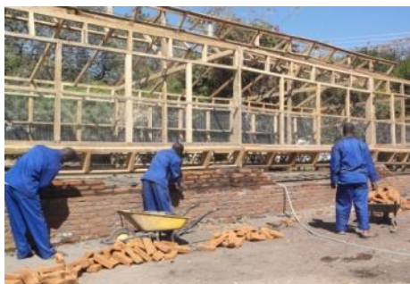
Fill in the gaps between the framework and the base/foundation with bricks.
