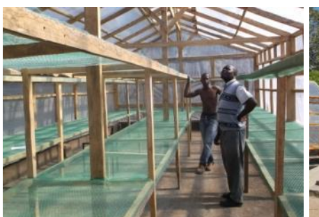
In the interior, build drying racks using 2"x 2" planks, chicken wire, and plastic gauze.
