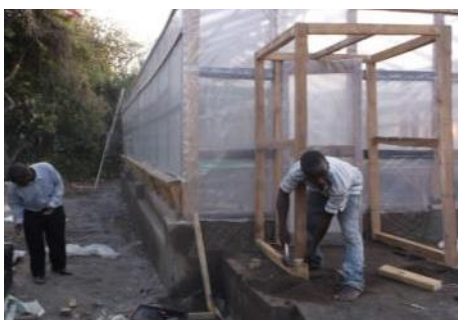
Finish by constructing a fly screening unit at the entrance/door.
